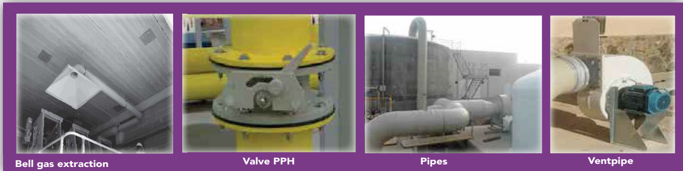
Bell gas extraction
