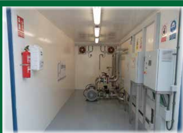
Biogas Combustion Plant, interior view
