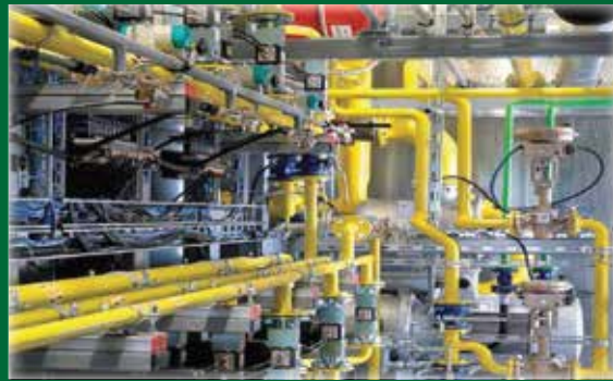
Interior view Biogas enrichment plant
