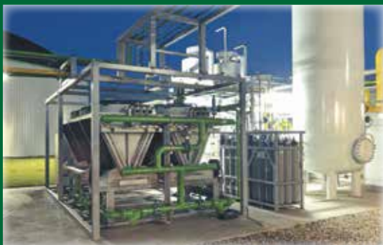
Biogas Upgrading Plants
