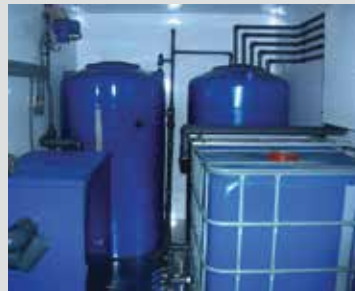
Pumping equipment 50m 3 / h
