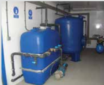
Filtration equipment 50m 3 / h
