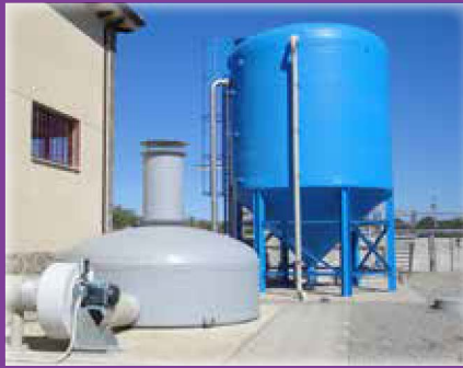
Deodorizing equipment 7000 m3 / h
