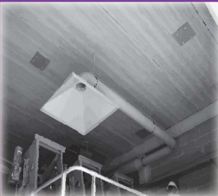
Bell gas extraction
