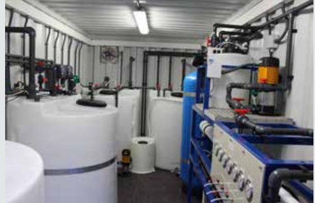
Interior of the Reverse Osmosis container
