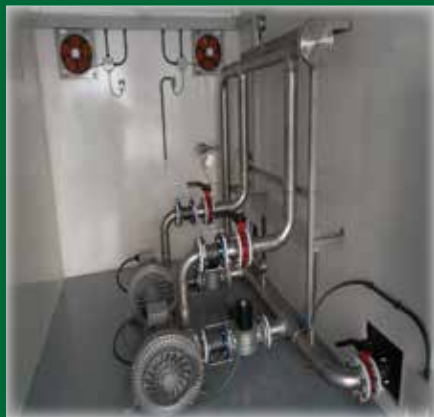
Biogas collection system
