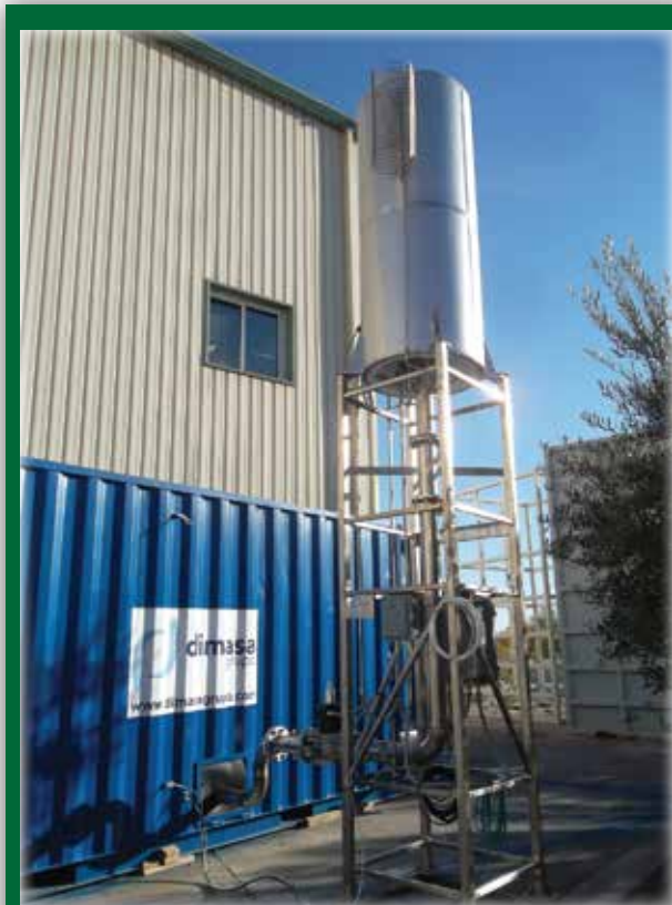
Biogas Combustion Plant, Exterior view
