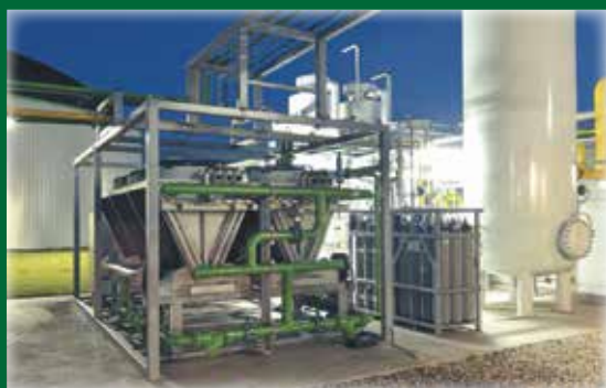
Biogas Upgrading Plants
