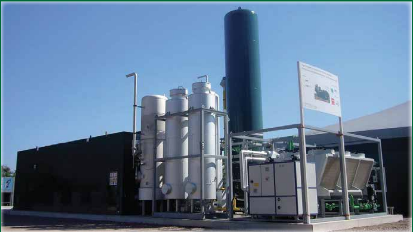
Biogas Upgrading Plants
