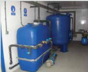
Filtration equipment 50m 3 / h
