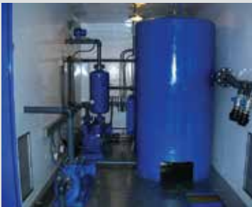
Vacuum equipment 350 m 3 / h
